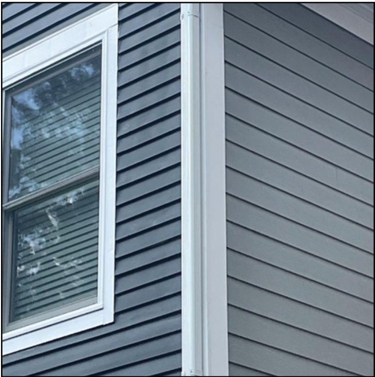
Left: Historic wood siding (left) and contemporary fiber cement siding (right) demonstrates the difference in overlap and thickness between the two types of siding.
